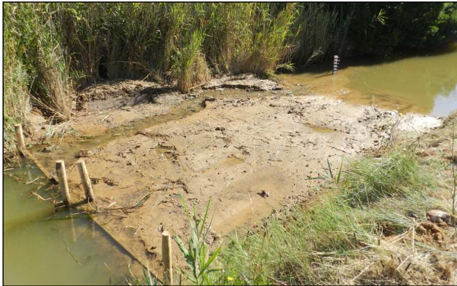
Barrage anti-sel renforcé
