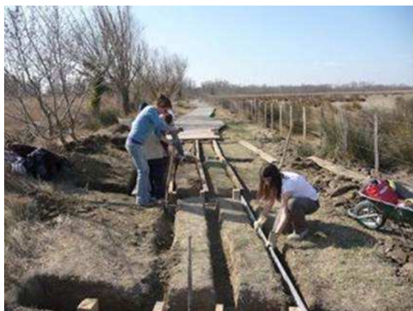
Figure 147 : Pose de bastings
