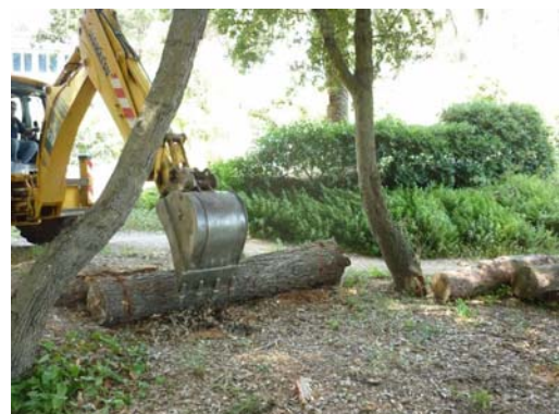
Installation de grumes anti-érosion
